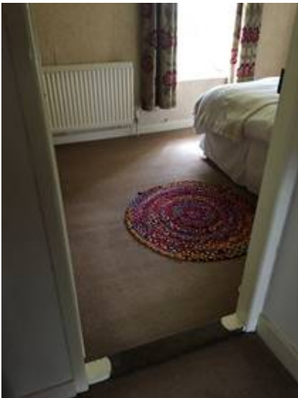
Entrance to the main bedroom, note the small threshold
